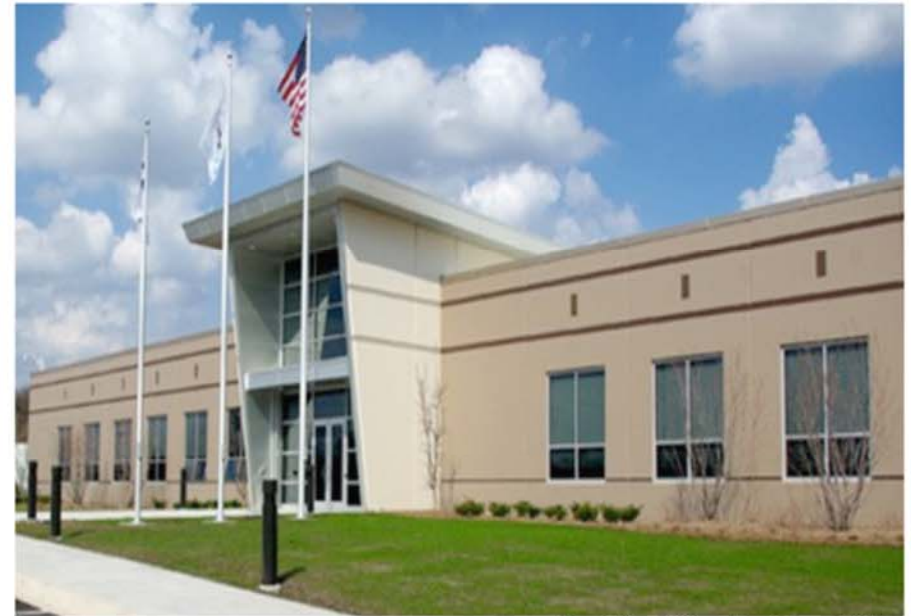
Public Works Facility
