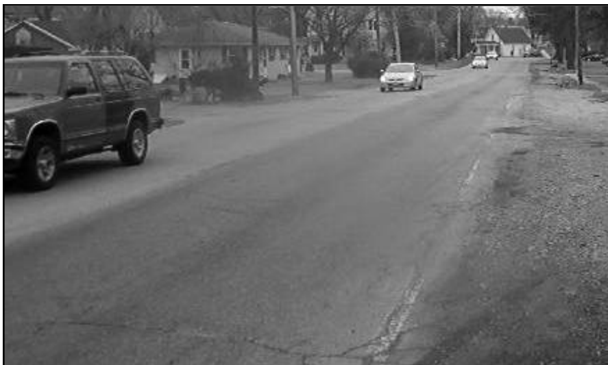
Williams Road from Lord Avenue to Washington Street is the final phase of the Lake Marian Road reconstruction project.
